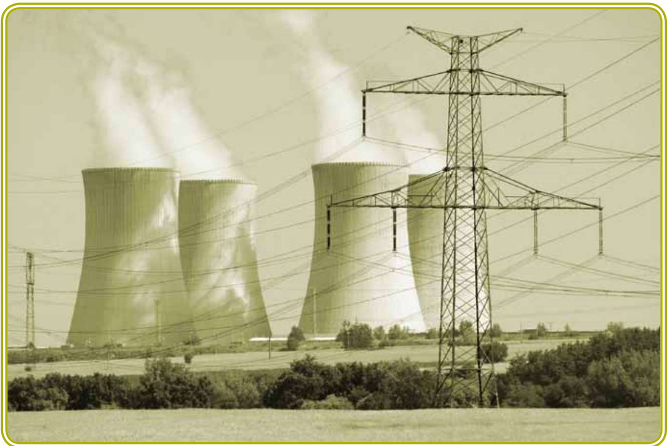
Nuclear power stations like this one are touted as a means to reduce carbon emissions.
