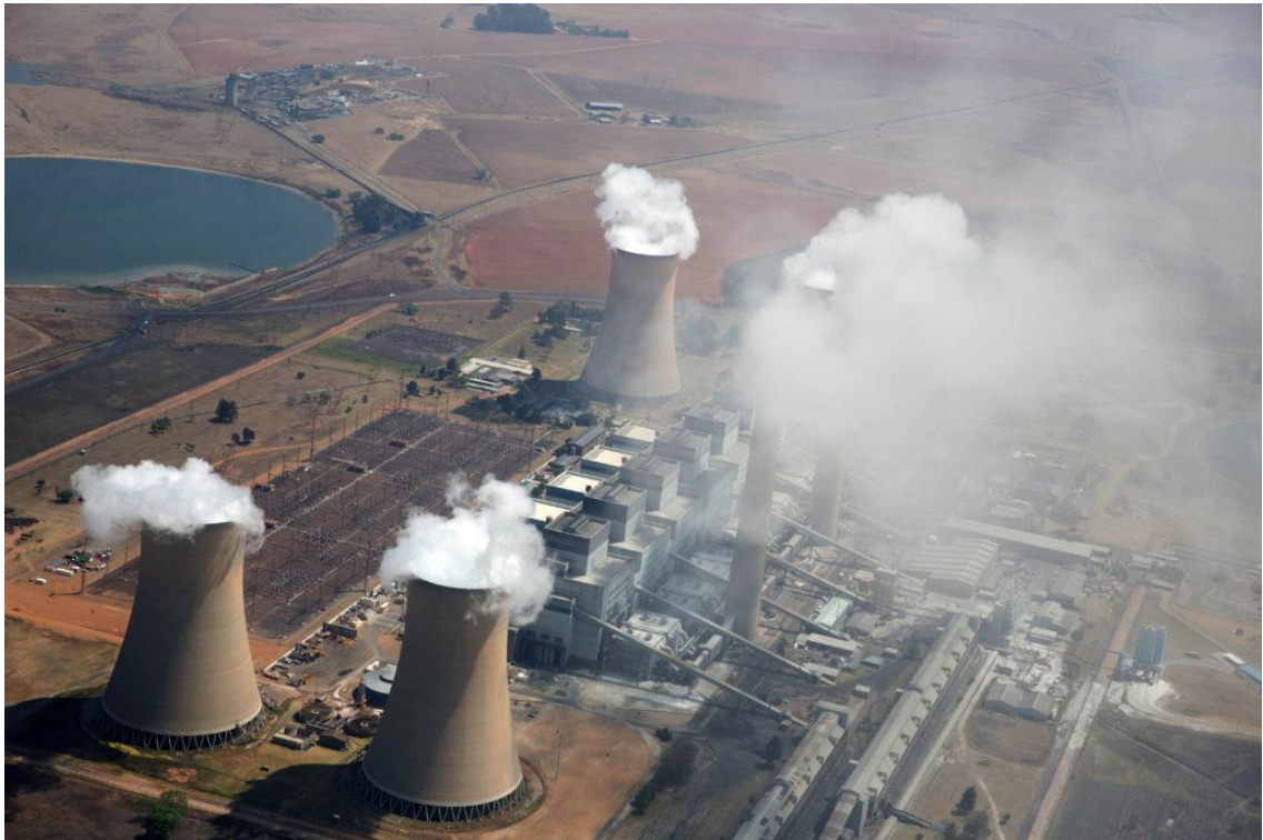
Kriel Power Station. Emissions from Eskom's coal-fired power stations cause significant numbers of respiratory hospital admissions and deaths. Image: James Oatway / CER
