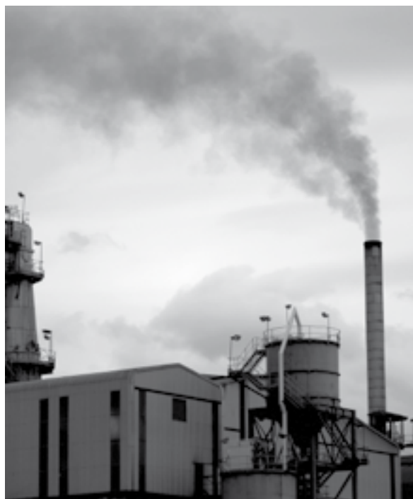
The Mozal aluminium smelter located 17 kilometres from Maputo in Mozambique. Photo by Zeca Ribeiro.
