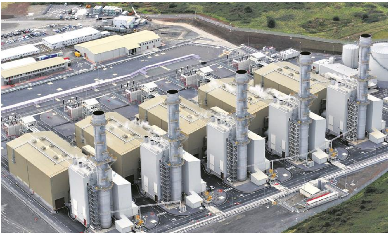
The Pembroke power station in Wales, similar to the one planned for Richards Bay
